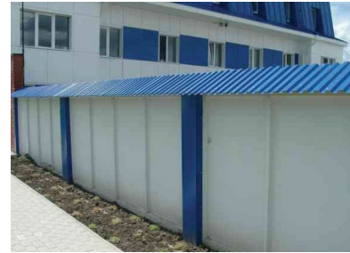
Pic.12 PUSH-TOP CANOPY OVER SOLID FENCE
